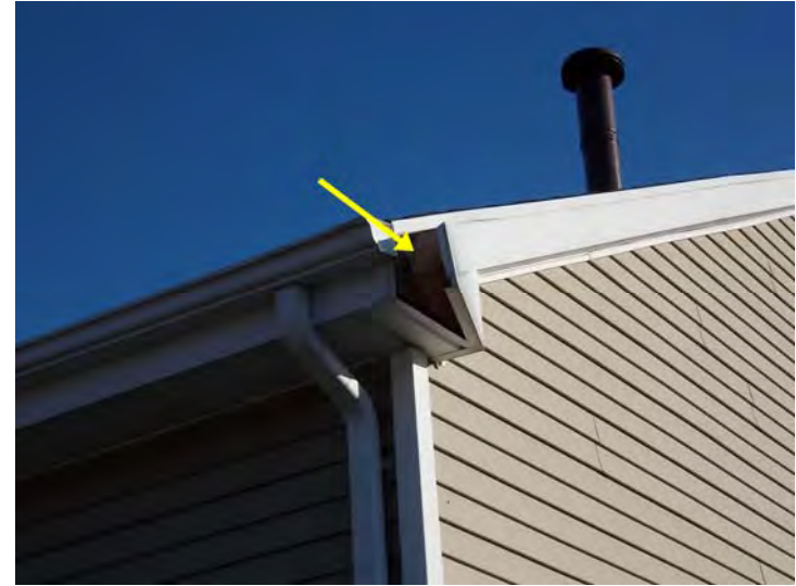
This trim section (on the community building) needs to be reattached to the building.
