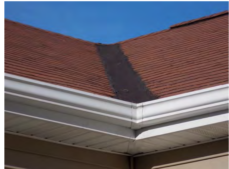
A tar-like substance has been applied to this roof's valley.
