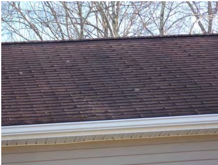
Roof shingles that are just starting to show signs of curling.
