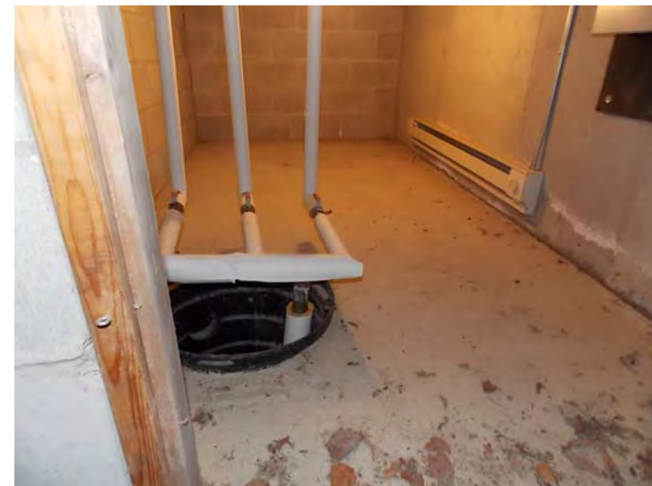
A typical domestic water distribution within the crawlspace of one of the residential building
