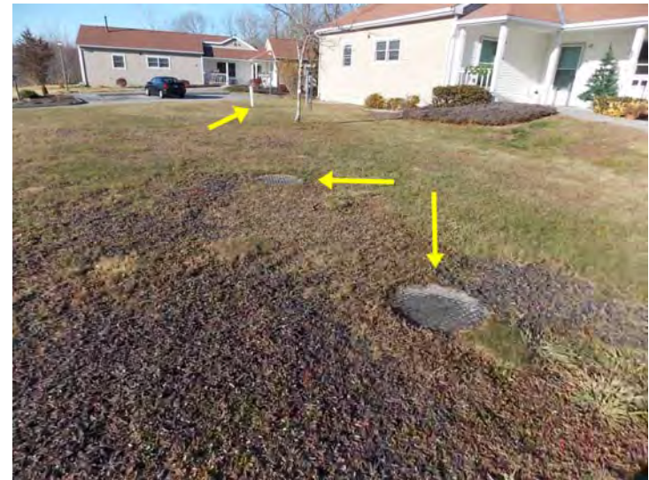
A pair of leaching field manhole covers and a vent pipe (arrows) near one of the residential buildings.
