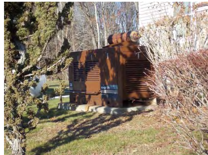
This generator provides emergency power for the community building and the domestic water supply system.
