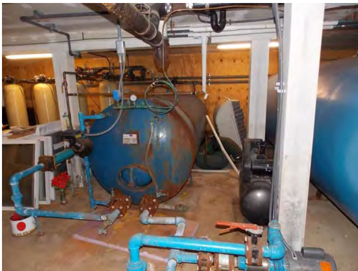
The existing domestic water system includes filtration (far left rear), pressurized supply tank (center) and a pair of 3,000 gallon storage tanks (portion shown on far right).
