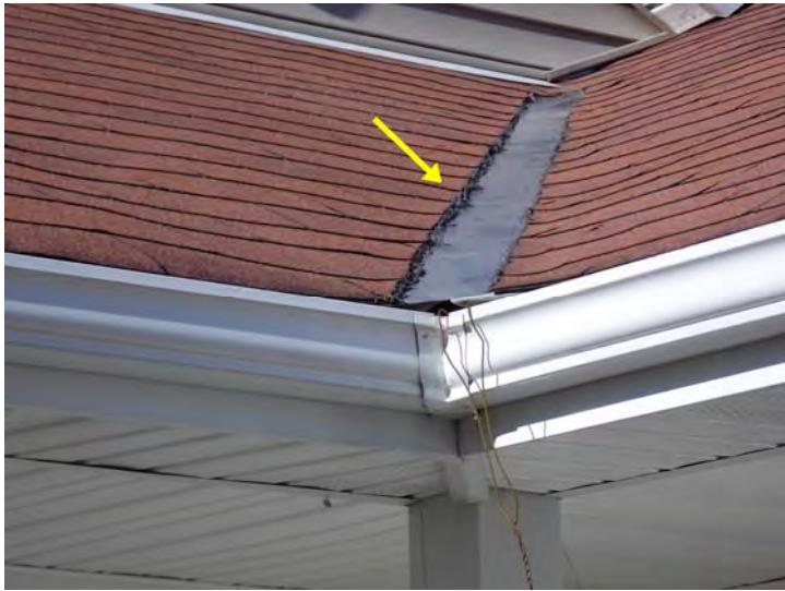
This roof's valley appears to have been covered with Plexiglas.
