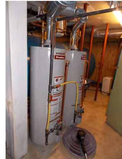
These are the propane-fired DHW tanks in the community building.
