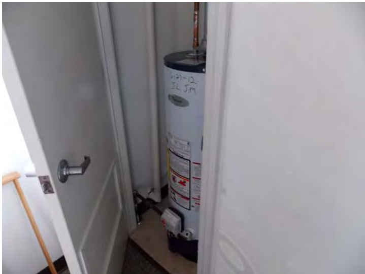
Propane-fired DHW tanks are located within a utility closet in each apartment.
