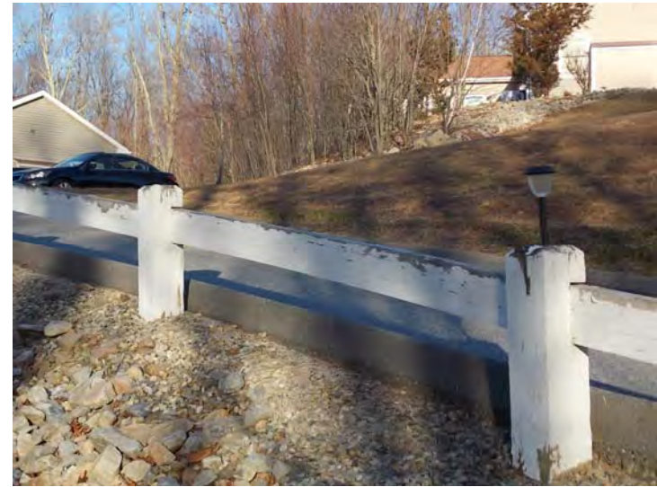
This driveway railing should be repainted.
