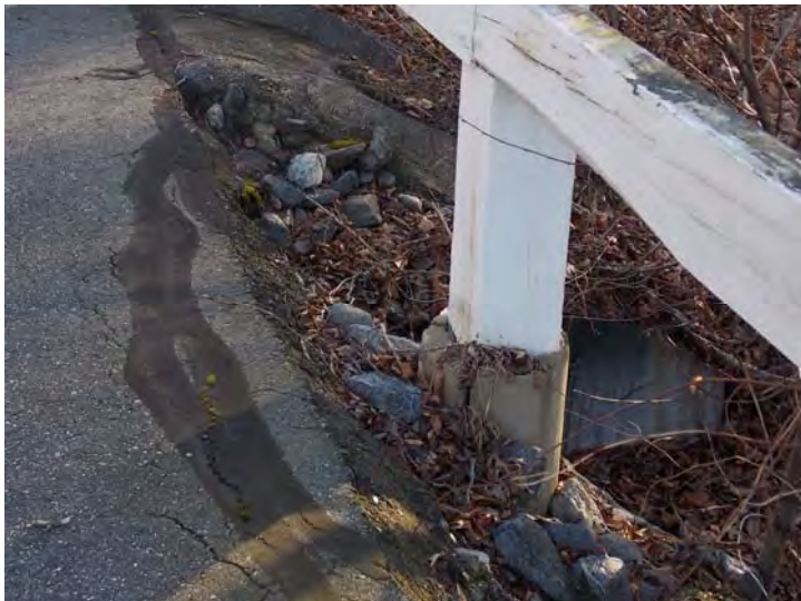
A close-up of a loose fence post and roadway damage at one of the bridge sections.
