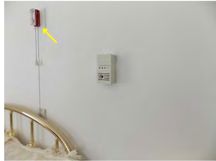
This apartment has a horn/strobe (arrow) and an older carbon monoxide detector.
