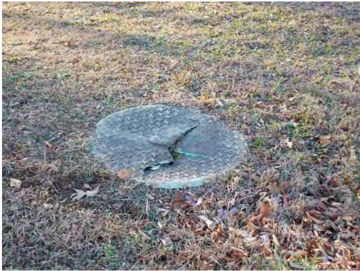
A recently damaged manhole cover. Repair from operating.
