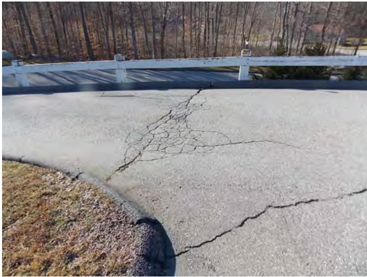
An example of a cracked section of asphalt paving.
