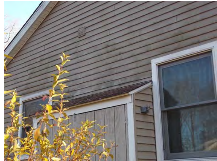
A vinyl siding section that should be power washed.
