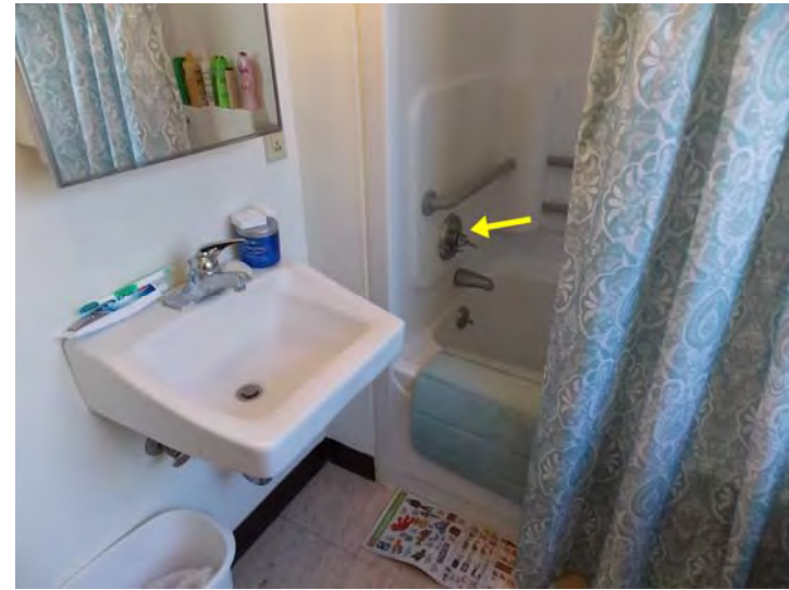
Bathrooms include an anti-scald mixing valve at the tub/shower.
