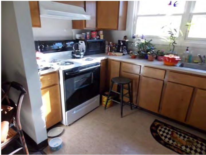
Kitchens have plywood cabinets, electric ranges, and VCT floor covering.
